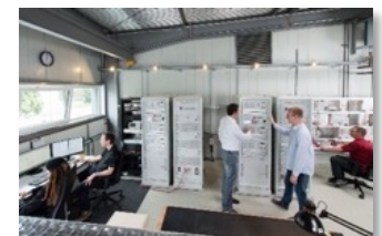
Power Hardware in the Loop (PHIL)
